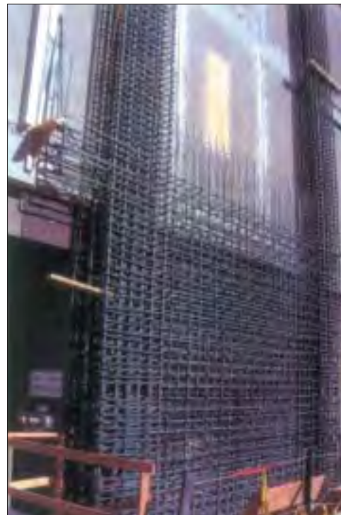
High volume Fly Ash has been used in the Barker Hall Project, University of California at Berkeley for the construction of shearwalls.
