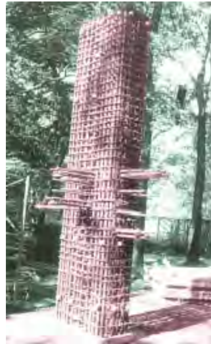
If this is the situation, what else is possible except self compacting concrete ? Above shows the mock-up trial of SCC at Kaiga Nuclear Power Project, (Karnataka).
