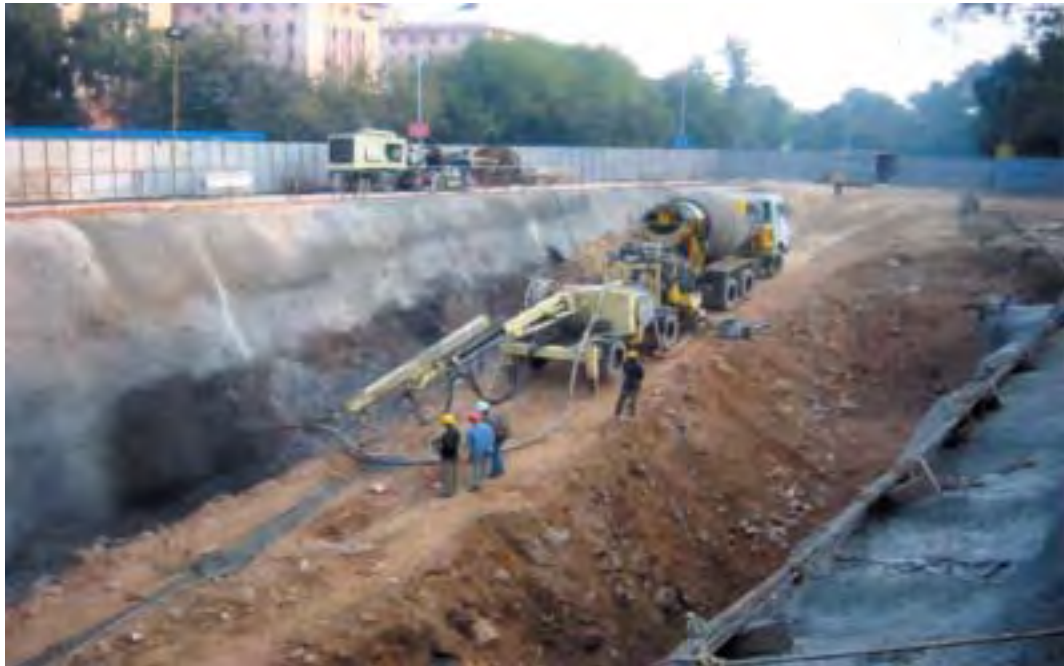
Shotcreting for slope protection by Robot Jet Machine at central secretariat, Delhi Metro.
