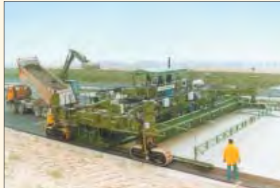
Fully automatic construction of concrete pavement.
