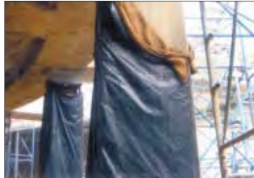
Curing vertical surface by wet covering.
