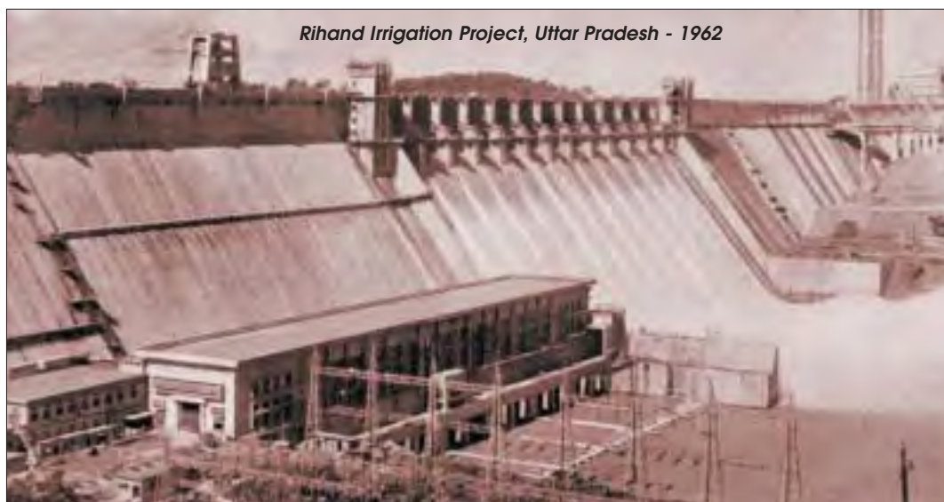
In India, fly ash was used for the first time in the construction of Rihand Project, Uttar Pradesh in 1962, replacing cement upto about 15 per cent.
