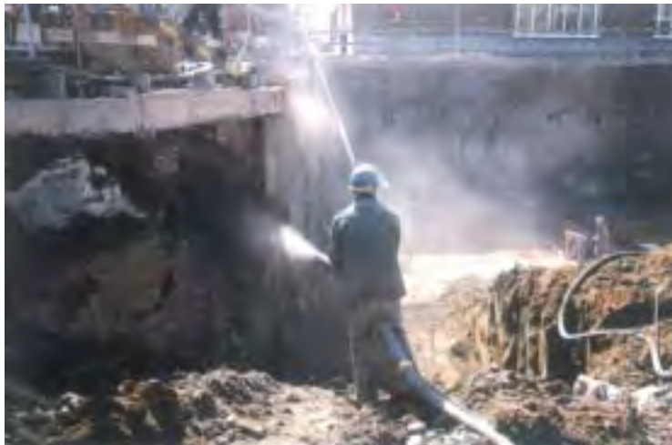
Steel wire fibre reinforced shotcrete
