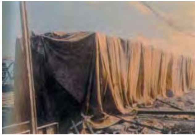
Beam under steam curing.
