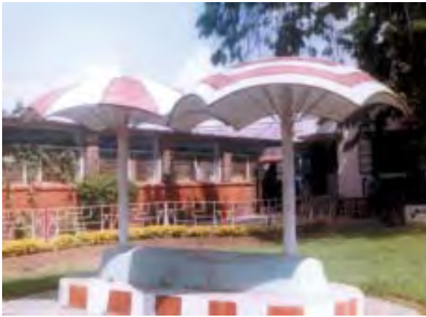
Ferrocement garden umbrella thickness 20 mm.
