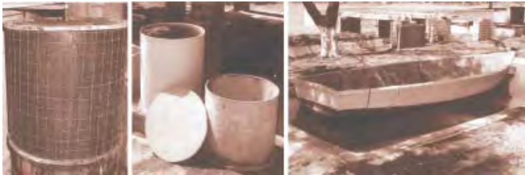
Small diameter wires and chickenwire mesh reinforcement used in casting ferrocement water tank
