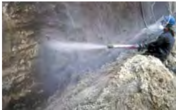
Shotcreting with steel reinforcement for slope protection.
