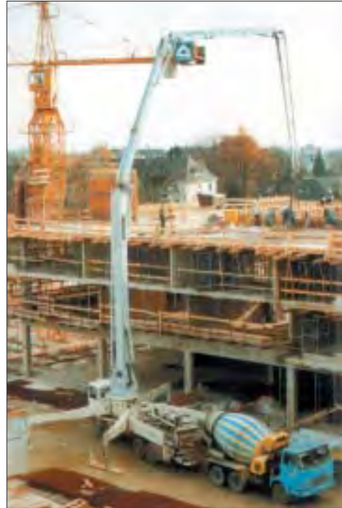
Placing concrete by pump and placing boom.
