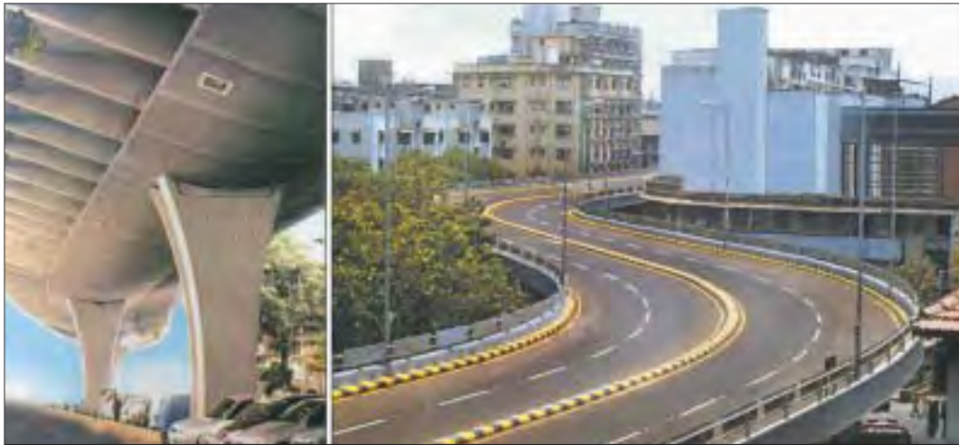
J.J Flyover at Mumbai where high strength, high performance concrete 75 MPa was used for the first time in India (2002).
