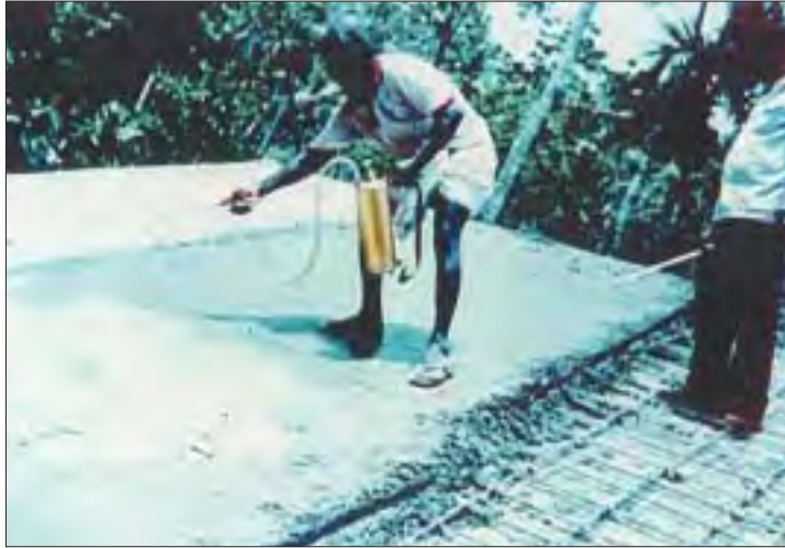
Membrane curing by spraying.
