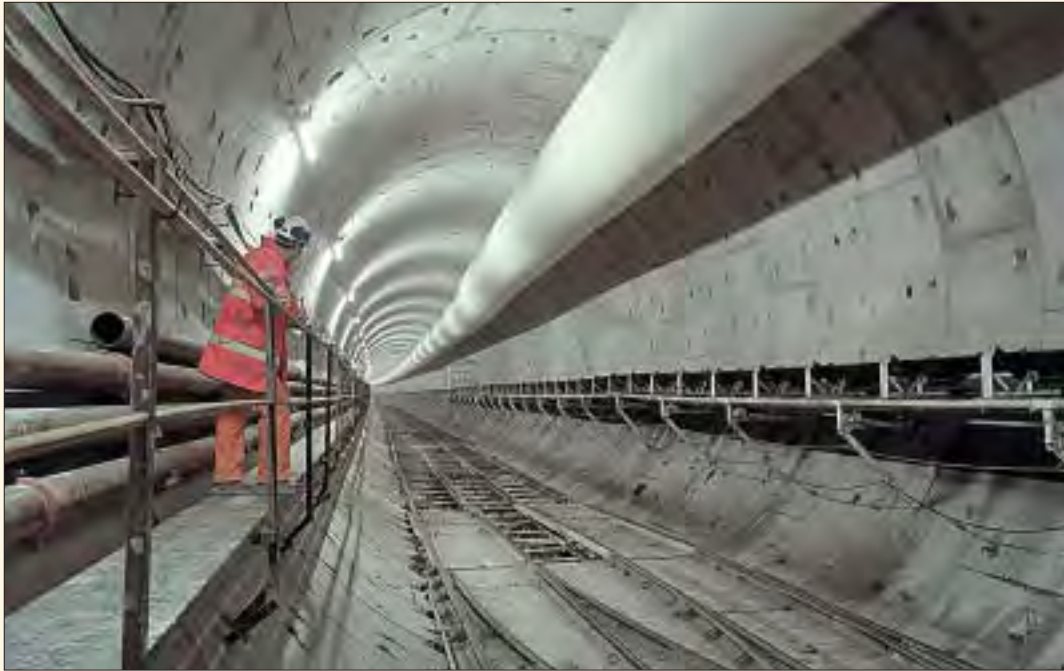
▲ CHANNEL TUNNEL RAIL LINK (UK). Tunnel diameter : 6.84 m and 8.15 m. Number of segments 9+key. Segment thickness : 350 mm. Concrete grade : 60 MPa. Dramix steel fibre reinforcement is used for casting segments without conventional steel.
