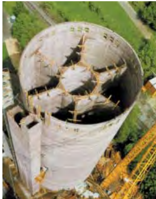
Cross section of multi-compartment silo.
